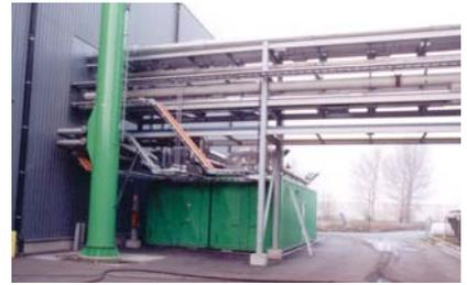
**Generated biogas is sent to the combined heat and power station. About 140 million cubic feet of biogas will be produced annually at the site.**
